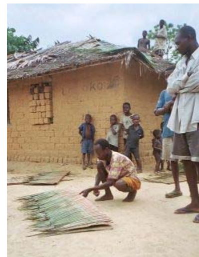
Figure 3. Using palm thatch to patch a hut roof. (Photo by Rick Alexander)
